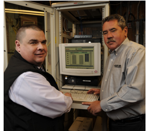
Scott Weber of Brookhaven Memorial, at left, and Chris Gibbons of Black Box Network Services, with the Toshiba Strata CIX1200 and Toshiba Network eManager. Using Toshiba Network eManager, Scott can remotely manage the entire telephone system from his desk.
